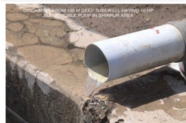
DISCHARGE OF WATER FROM 100M DEEP TUBEWELL HAVING 10 HP SUBMERSIBLE PUMP IN SHIRPUR AREA
