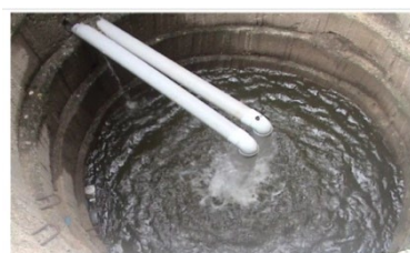
Figure.5. Artificial recharge through the dry dug well in alluvial area of shirpur taluka
